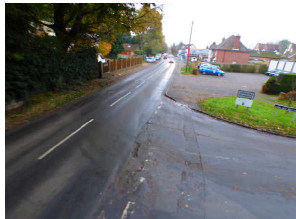
A clear change in the speed profile and character needed from this point
